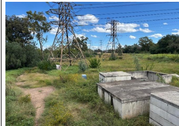
Plate 6: Phase 2 Sludge Pipeline Route End Point
